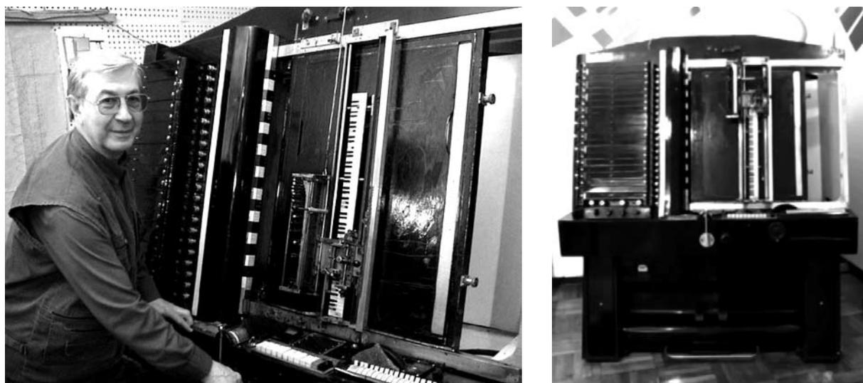
built in 1964, contained 720 pure tones covering the range of 21 hertz – 21.6 kilohertz (covering 10 octaves), with five optical discs with oscillation speed of respectively 24, 6, 4/4, 6/16 and 6/64 rotations per second.
